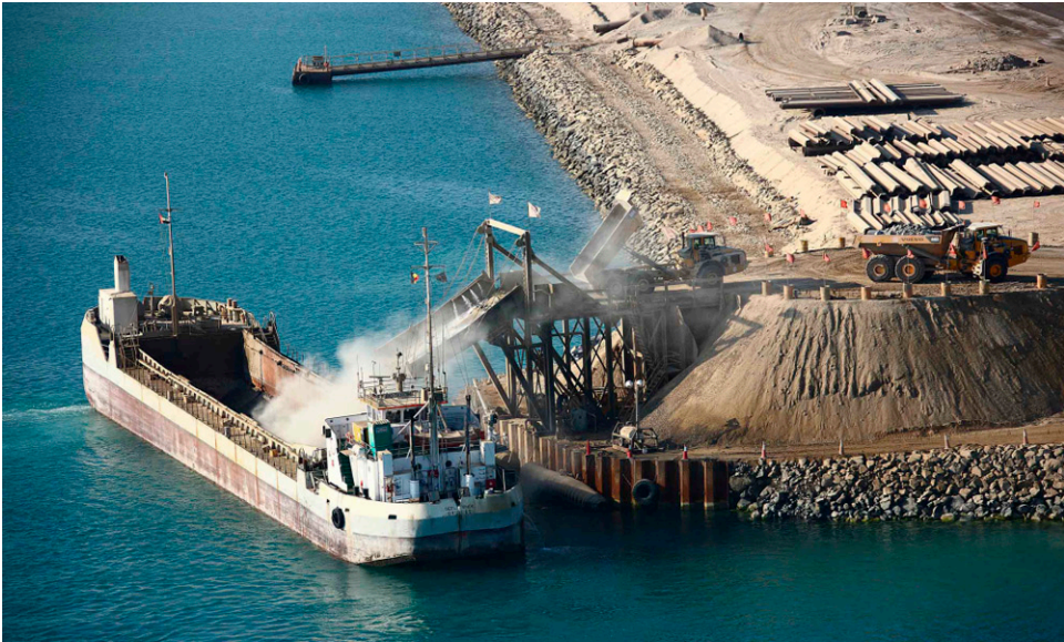
Figure 7. Aerial view of jumbo-sized dredgers filled with rocks for The World breakwater formation, April 2008. Source: Courtesy of Nakheel.
